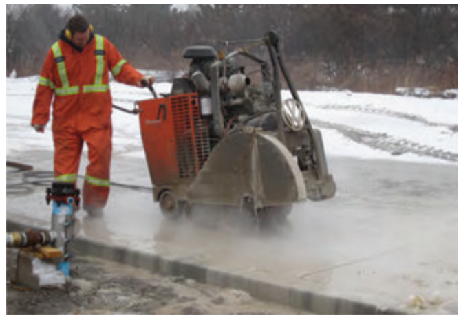
Sawcutting concrete pavement.
