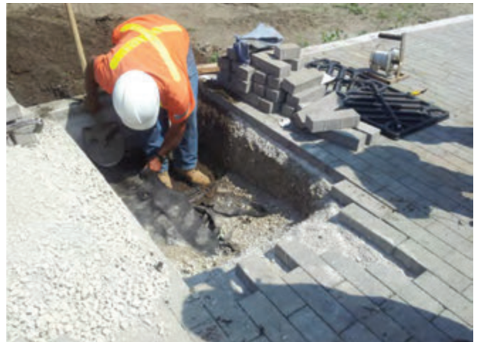
Cover over the cell deck with the cut geotextile and add an overlapping layer of geotextile on top.
