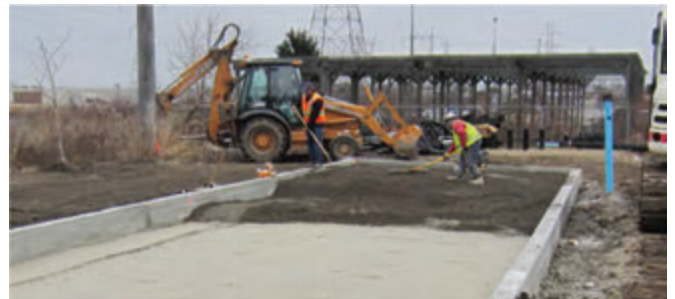
Backfill installation on top of deck.
