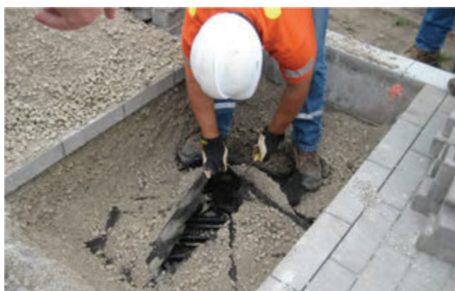
Geotextile is cut through centre of cell deck.
