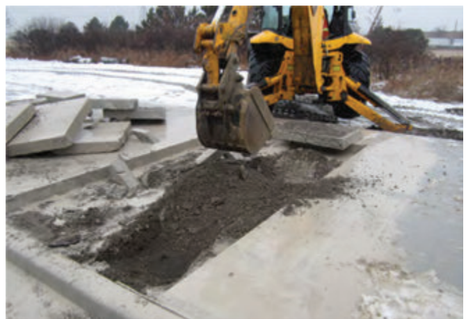
Mechanical removal of pavement to expose soil cell decking system.
