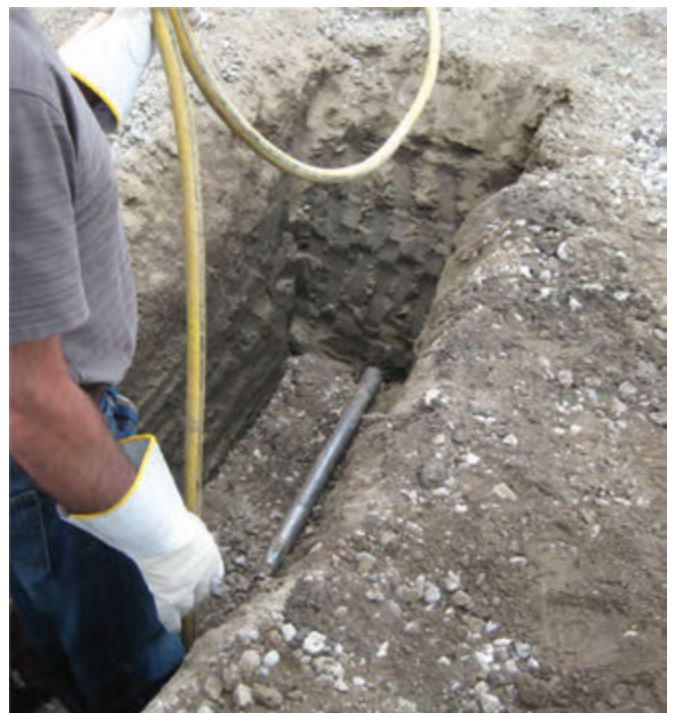
After false start on imaginary building end, torpedo is reset at road end.
