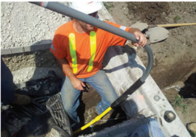
Riser is attached and pulled through.
