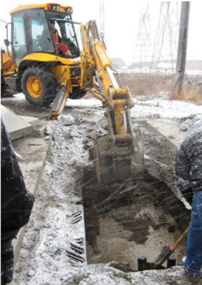
Mechanical removal of soil cells.
