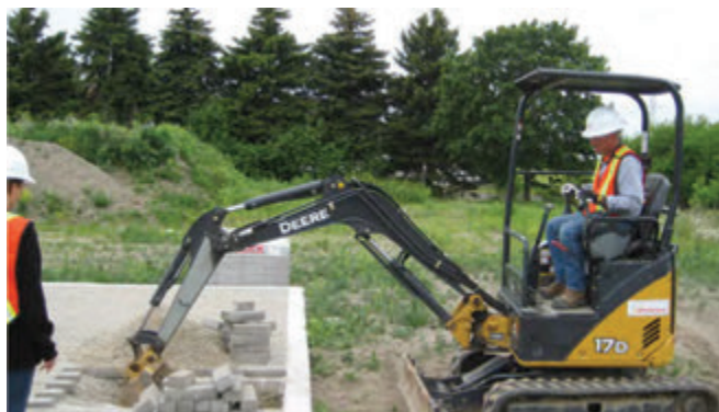
Removal of pavers and granular base.
